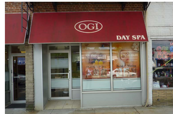
Examples of storefronts on Main Street that include recessed entrances, maximize window displays and avoid excessive signage
