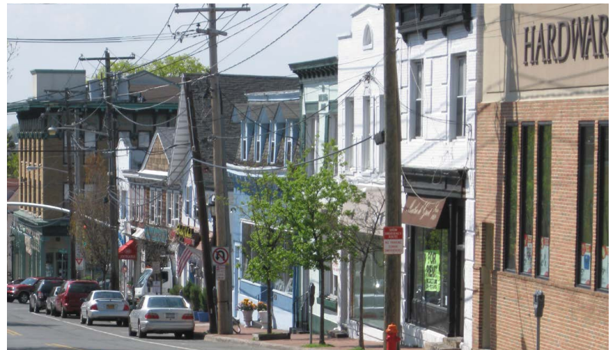
Differing facade finishes and colors
